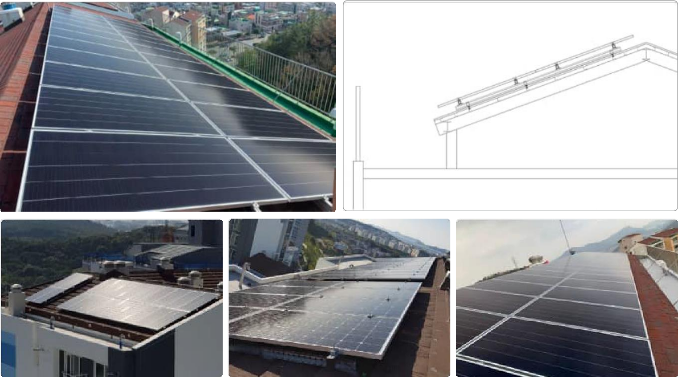
Access inclined roof photovoltaic generation device is for inclined roofs of LH apartments and inclined roofs of public facilities, and is a system that can satisfy both efficiency and aesthetics with an integrated installation method with the roof inclination angle. It is a rail-type construction in which the support is not exposed to the top.
