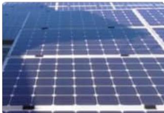
Deterioration of power generation performance (shade, aging)
